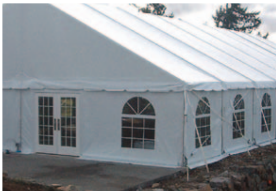
Window Wall and Double Glass Doors
